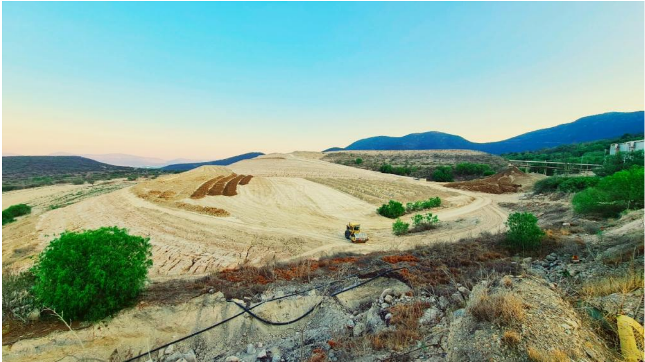
Figure 13-3: Dry tailings being collected and hauled to the tailings pond
