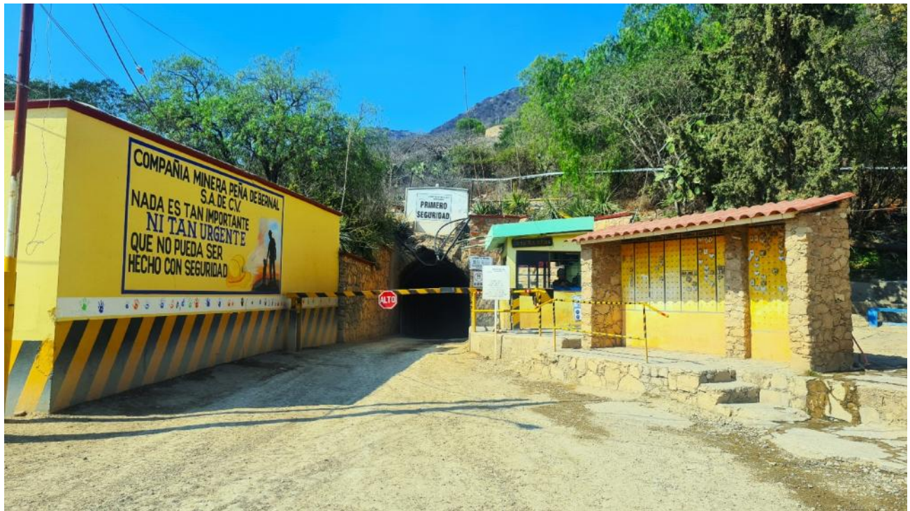
Figure 18-2: Portal of the incline for access to the San Martin mine
