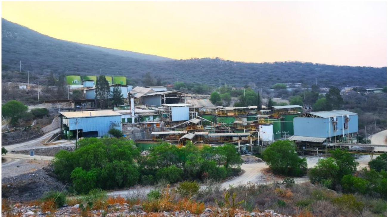
Figure 13-2: General view of the process plant at San Martin
