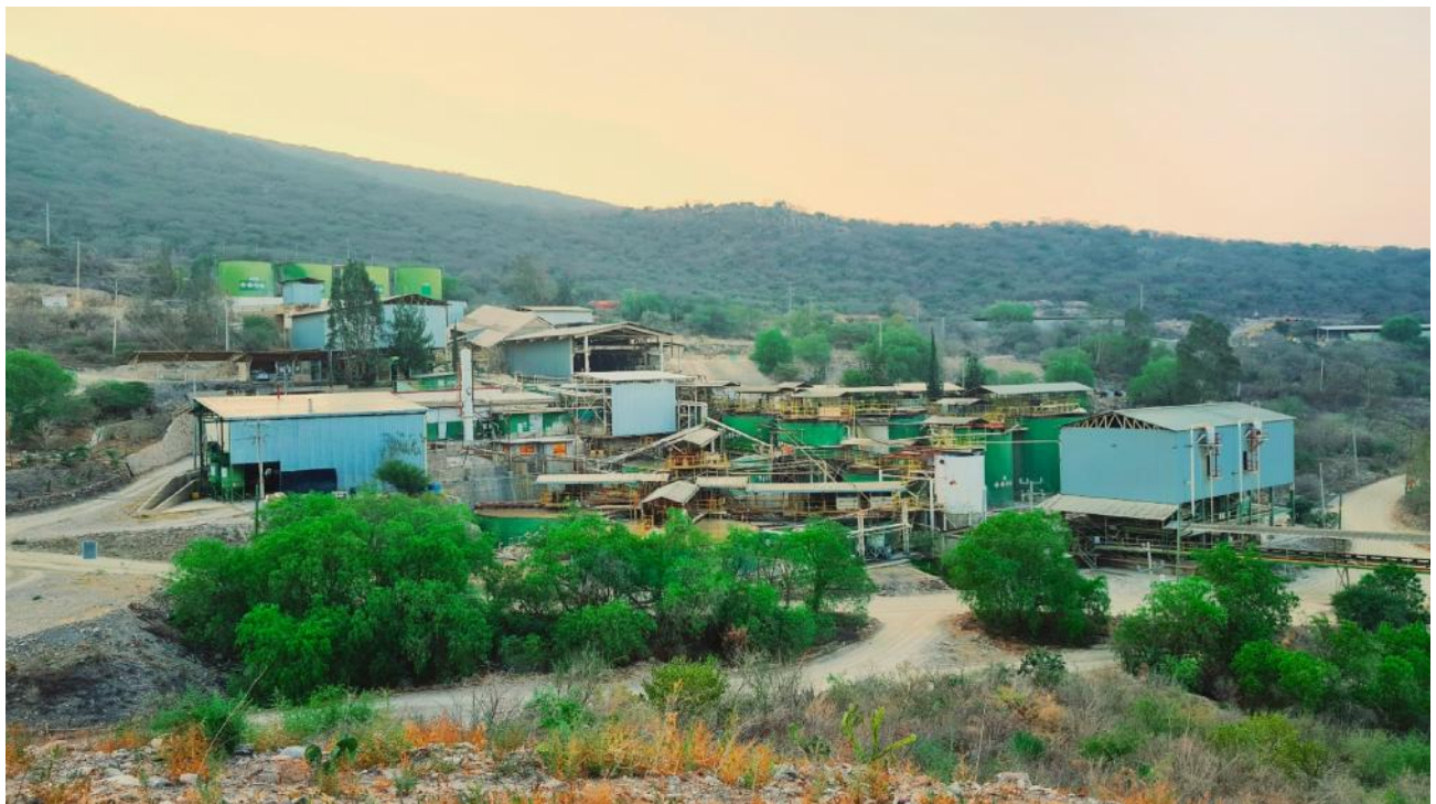
Figure 18-3: General view of the processing plant at San Martin
